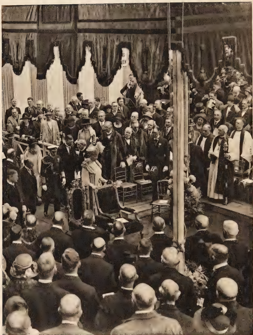
H. M. The King laying the Foundation Stone of Lloyd's New Building 23. May 1925
